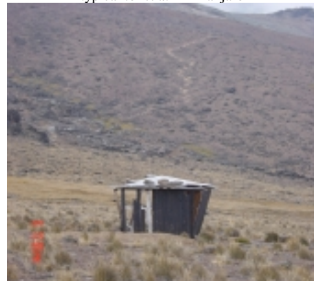
typical toilet at Kilimanjaro
